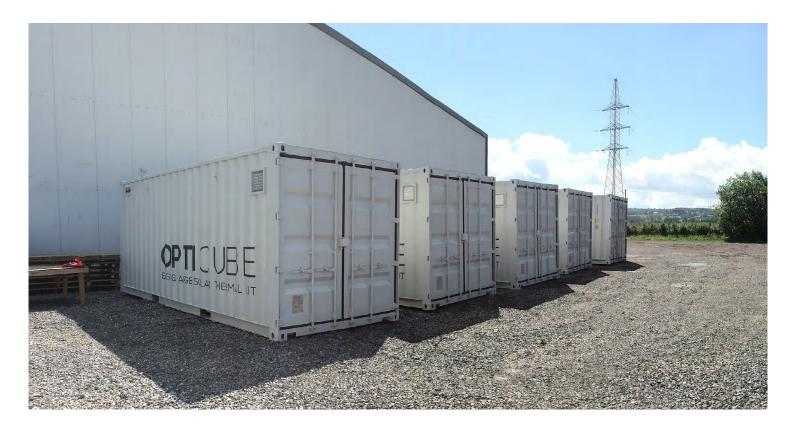
The Opticube Field concept starts around a 40 foot double door container (one on each side). It is then modified and equipped in the workshop to meet the needs of the customer. This way, the container is transformed into a real heating room. But before describing the hydraulics of the installation, it is important to review the equipment that is not directly part of the process but that also has all its importance in a boiler room.
